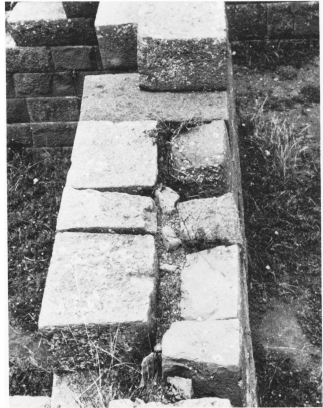
Fig. 33. Sometimes the building blocks were fitted only along a shallow band close to the visible face of the wall, while the interior of the joints was filled with rubble.
