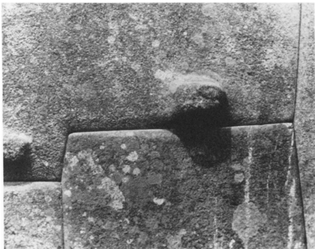
Fig. 28. Exception to bedding-joint rule at Ollantaytambo.
