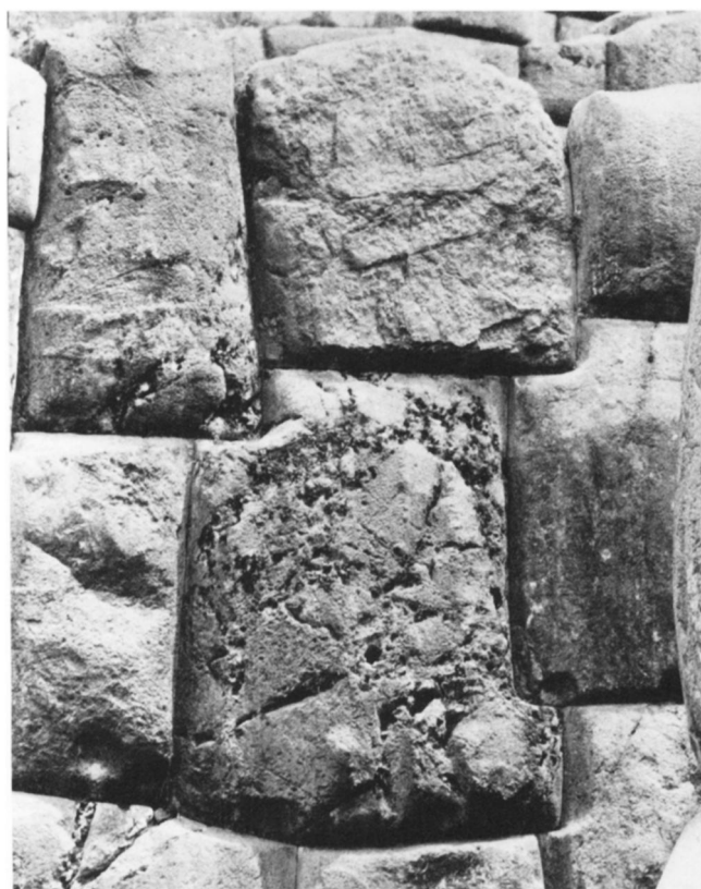
Fig. 35. Illustration of the combined effect of the fitting of bedding joints and lateral joints at Saqsaywaman.
