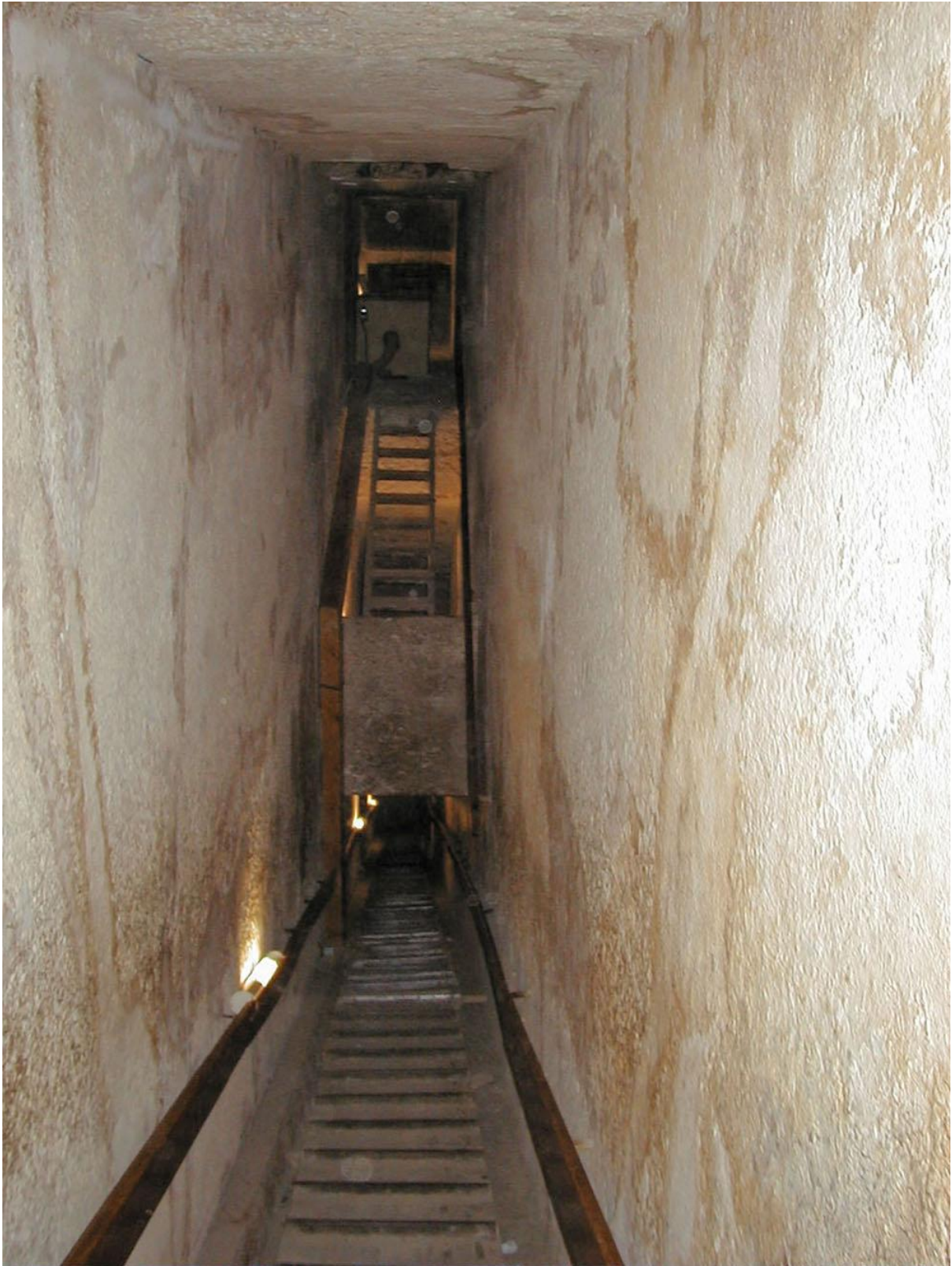
Looking north from the horizontal passage, showing the lower inclined passage, which is the route tourists take today; the upper entrance passage and the lower chamber are off limits.
